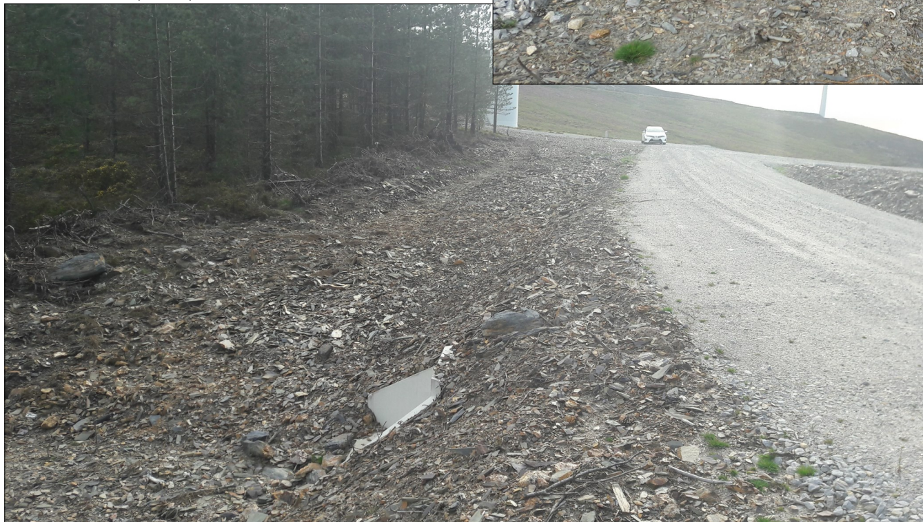
Foto 3—Acesso (talude) vista do AG
